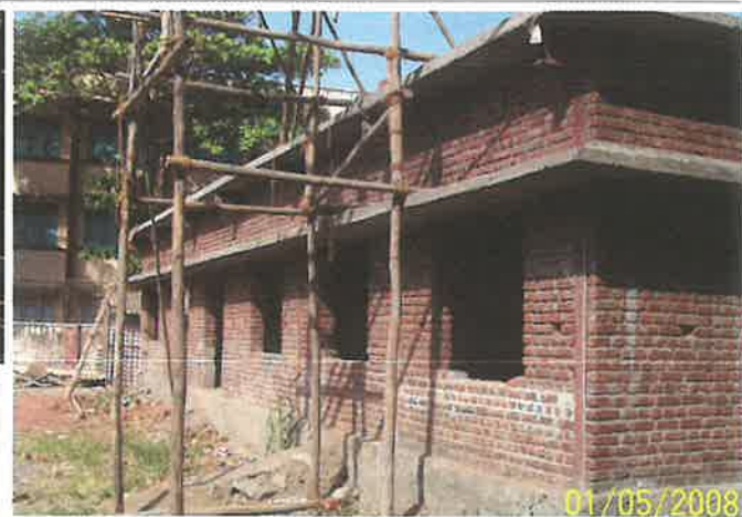
Looking towards west, construction of buddhist community hall, municipal school
