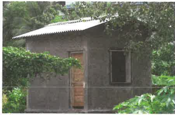
Cabin under construction
