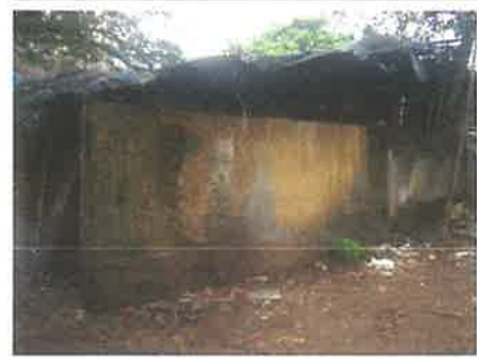
Workshop on southern side
