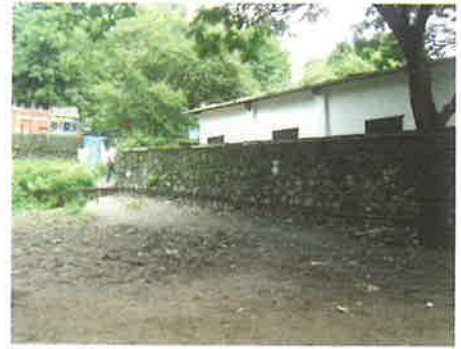
Encroachment - private gym
