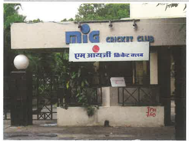
Main entrance gate
