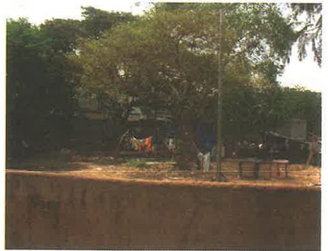
Dividing wall and encroached part
