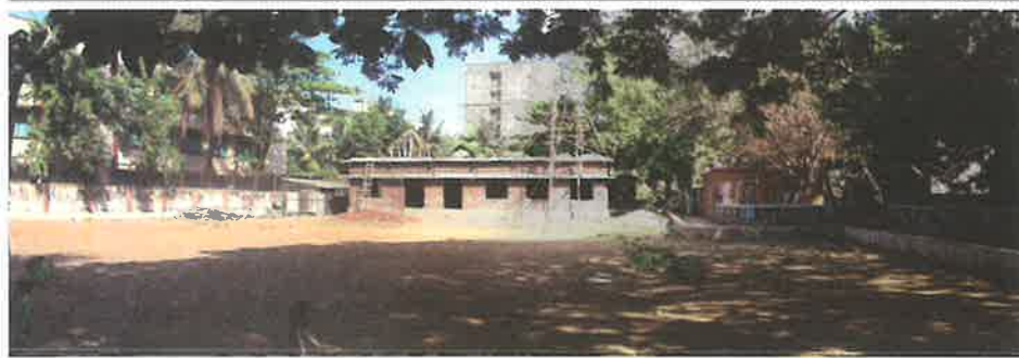
Looking towards west and northwest, construction of buddhist community hall
